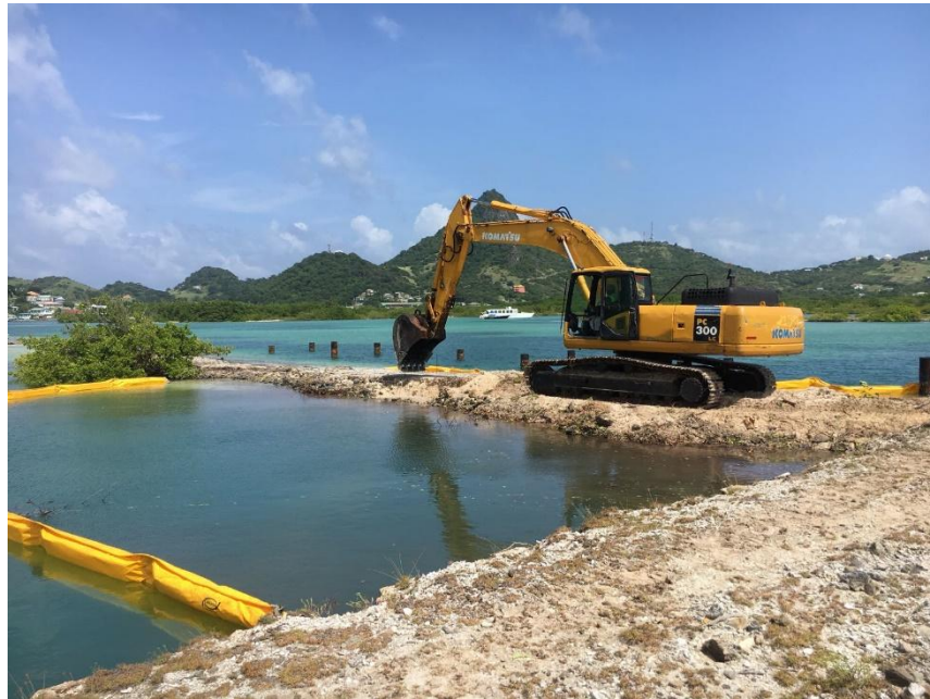
Excavator beginning work on Pier#2
