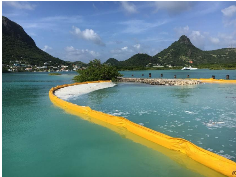
Turbidity barriers put in place for excavation.
